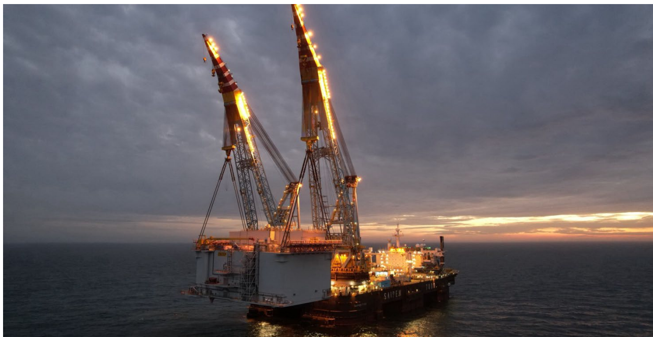
Fig 6: Second HVDC offshore platform being installed at Dogger Bank B
